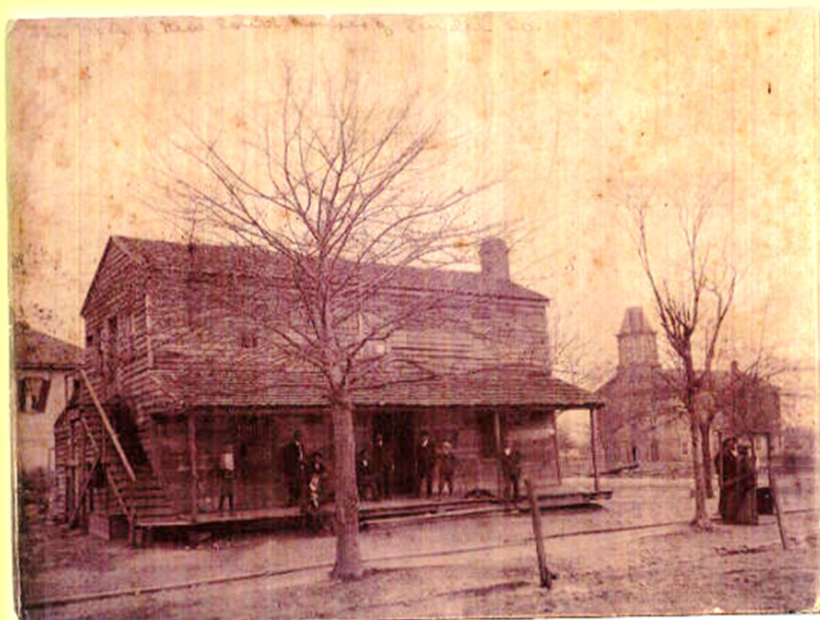
Old and New Court House of Pender County
